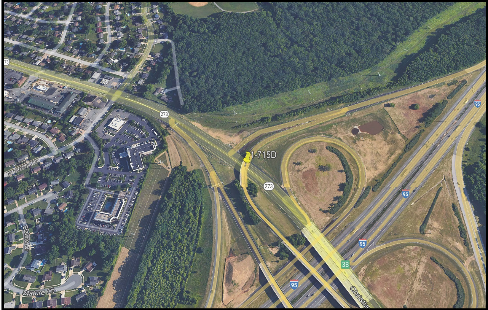
BR 1-715D (Ramp 6048 over SR 273)
