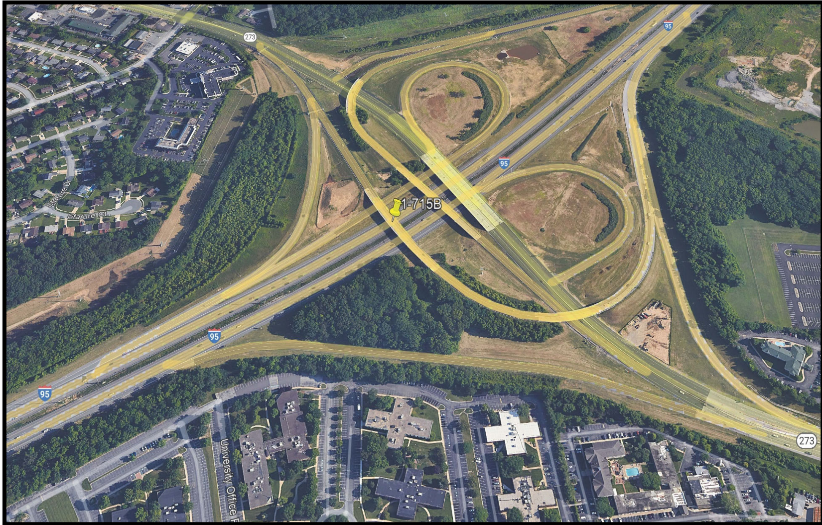
BR 1-715B (SR273 / I-95 Ramp over I-95)
