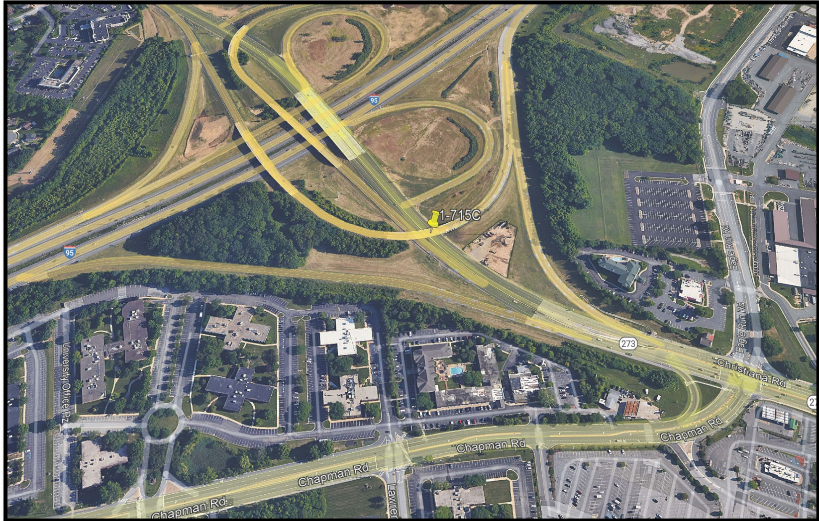
BR 1-715C (Ramp 6047 over SR 273 / Christiana Rd)
